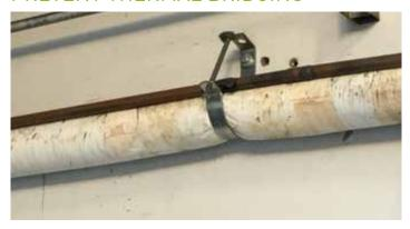
Insulation compression at suspension locations breaks the thermal barrier. This results in thermal bridging and could cause condensation, freezing points and mold growth.
